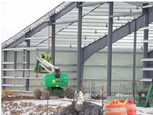
Crews work to build the Carrollton Field House.
